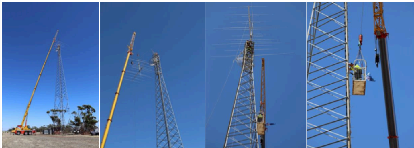
02Feb2026: A complex and carefully planned operation with a 70m crane
