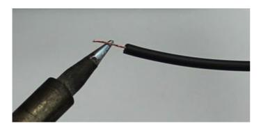
Keep the iron in place and touch the solder to the wire until it's fully coated. Repeat this process on the other wire.
